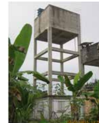
Elevated storage tanks of groundwater
